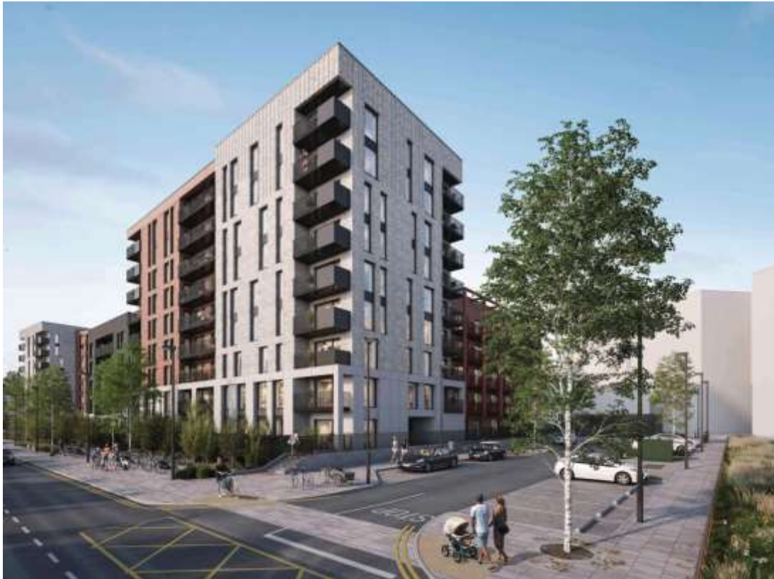
Figure 10 – CGI View of Proposed Development from Dyke Road
